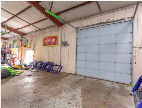
OVERHEAD DOOR ACCESS
