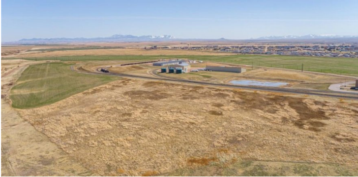
SITE LOOKING WEST
