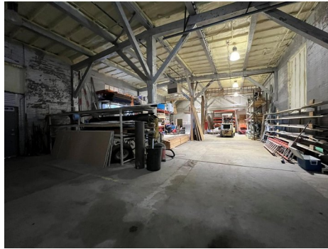
HEATED SHOP / WAREHOUSE BAY
