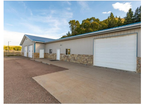
WAREHOUSE / SHOP EXTERIOR
