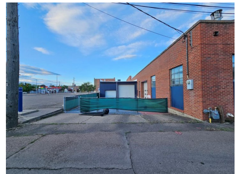
REAR DRIVE-DOOR ACCESS
