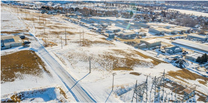
SITE AND ADJACENT SUBSTATION
