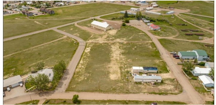
AERIAL TOWARD CUT BANK
